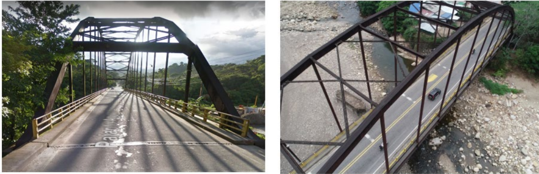
Figure 1. Unete bridge front picture and aerial view using a drone
