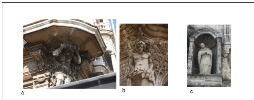
Figure 5. Sculptures located in Old Havana City affected by black crust and dust due to environmental pollution. a) Atlantes, Embassy of Spain. b) Atlantes, Cueto Palace. c) Saint Charles statue, Havana's Cathedral
