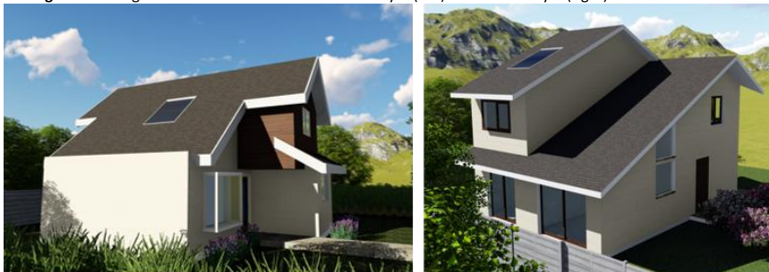
Figure 13. Integration of solar collectors in case study A (left) and case study B (right). Source: the author.
