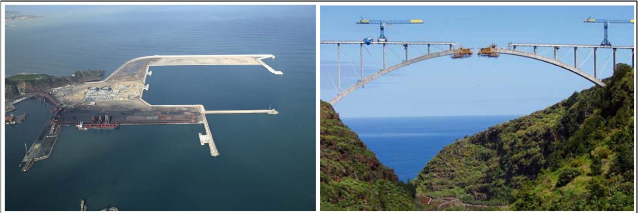
Figure 4. Conquest. Outer Port of Gijon (Asturias) and Los Tilos Viaduct (La Palma Island). Source: www.puertogijon.es , www.ferrovial.com
