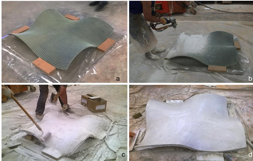
Figure 3. Manufacturing process of a GRC panel. a. Fixed mesh. b. GRC sprayed. c. Removing excess material. d. Trowelling and finish job. Source: Prepared by the authors.
