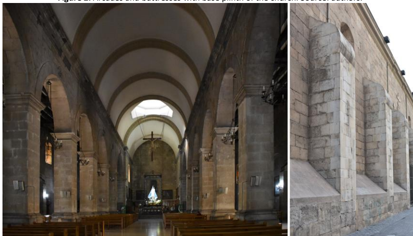
Figure 2. Arcades and buttresses with base plinth of the church. Source: authors.
